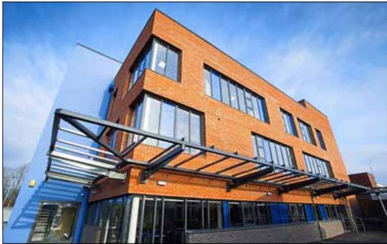
The new teaching block at St John Fisher RC High School, Staffordshire
